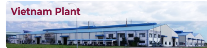
Vietnam Plant Vietnam Plant (Ho Chi Minh, Vietnam) · FCAW / SAW / GMAW Production
